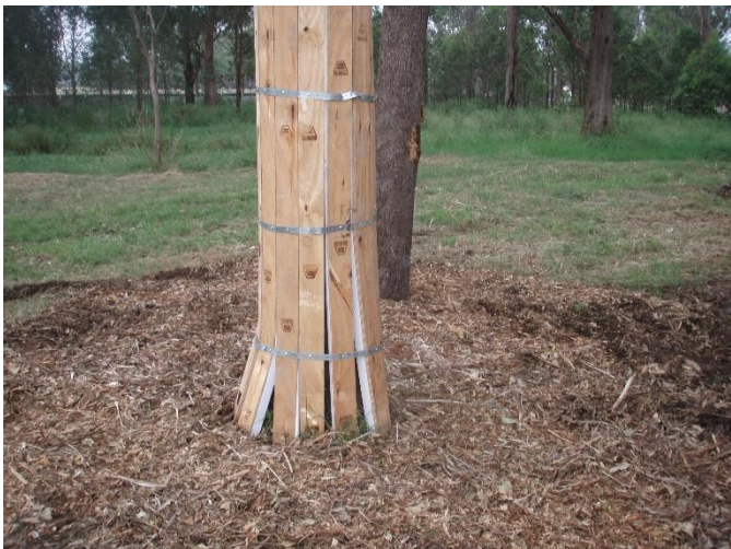
Photo 15: It is flexible for a better fit and attached using screws to avoid light impact.
